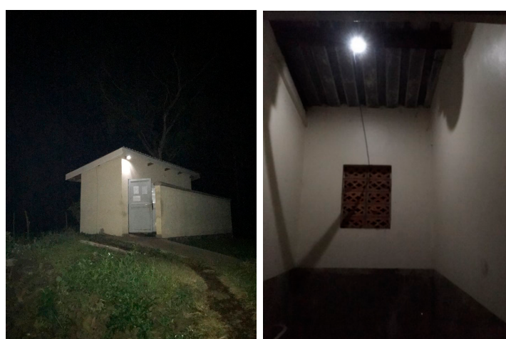
Figure 3. Photos of lights powered by the Pee Power system outside of a latrine block (left) and inside a toilet cubicle (right).
