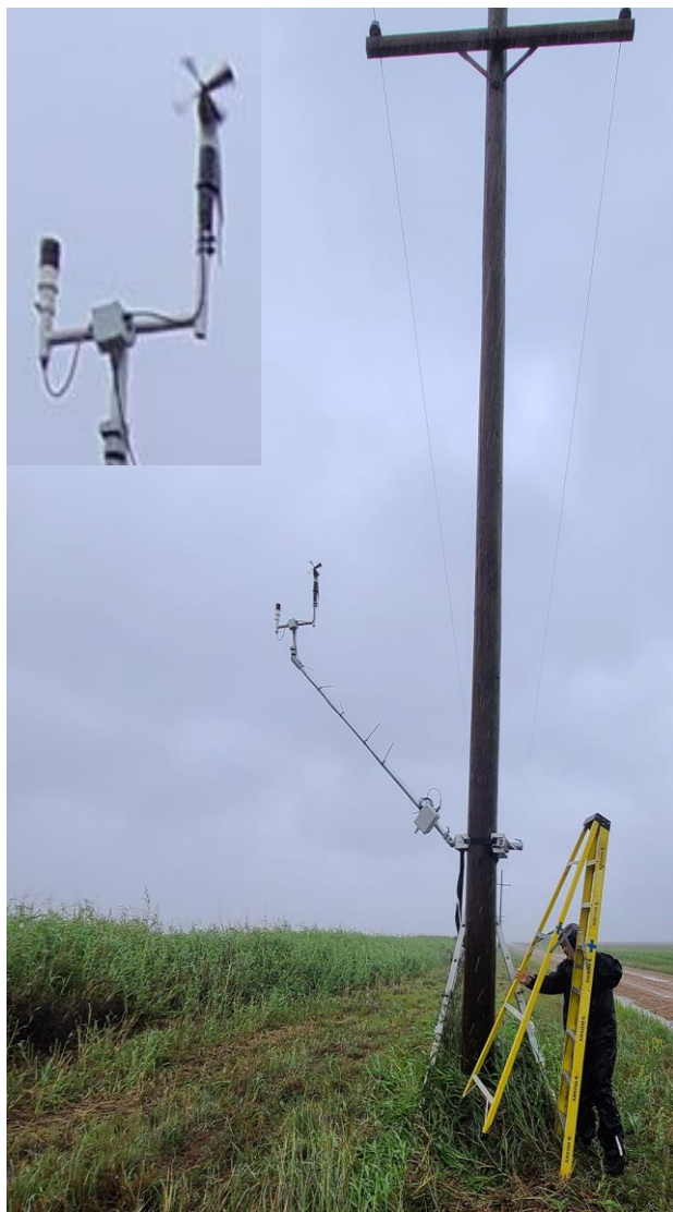
Figure 11. FARM POLENET unit being deployed on power pole during hurricane Delta (2020).
