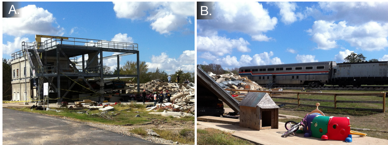
Figure 1: Photos taken during a visit to Disaster City training facility in College Station, Texas, USA. A. A collapsed structure prop used for training on different complex forms of search and rescue techniques such as shoring, breaching, bracing, and use of dog, and B. a train wreck prop is used for real-life drills and training on specialized SAR techniques, such as rescue in confined spaces. Using these props, responders can train on SAR techniques, such as conducting different physical search methods, using listening and visual devices, breaching concrete, and canine search training. (Photos taken by Z O. Toups).
