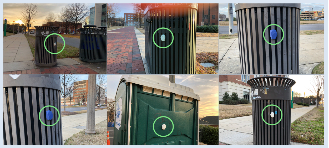
Fig. 5. Some samples of the installed beacons are at the study sites. The beacons in the circle are installed on the targeted amenities surface to localize them.
