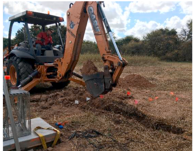
Fig. 8. Empty trench excavation.
