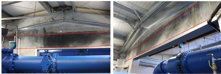
Figure 5. CFRP applied around the perimeter of the portal as denoted by red dotted lines.
