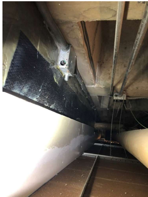
Figure 9. CFRP retrofit above ceiling grid covered by drywall panels at Boney Courthouse.
