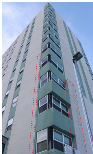
Figure 12. Boundary elements confined with EBFRR and bolts on MKT, marked by red dashed lines.
