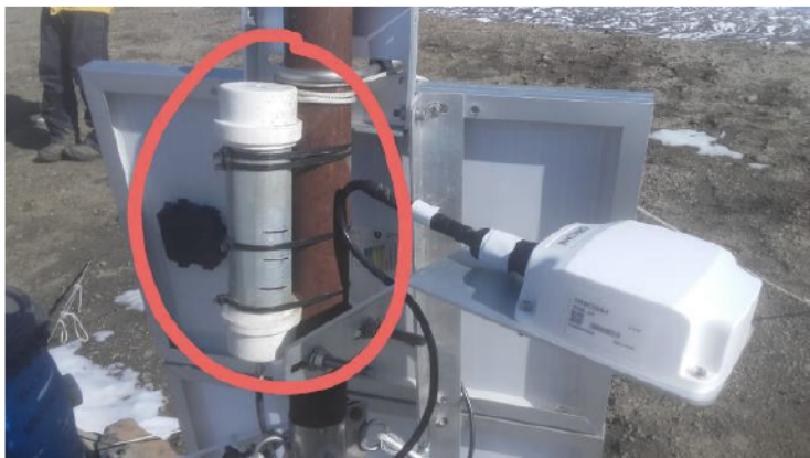
Figure 6. Closeup photograph of the Brazilian permafrost monitoring station on Seymour Island with the improvised radiation shield circled in red. The Campbell 107E temperature sensor is inside this shield. Photo by personnel from Marambio station, taken in February 2020.
