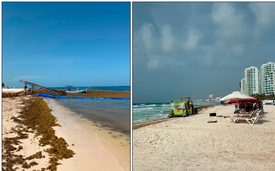
Figure 5. Seaweed is removed from beaches in the Riviera Maya using a variety of techniques, such as the blue floating booms used by the city of Puerto Morelos (left) and tractors with sweepers used on the beaches of Cancun (right). (Photos by C. Gallaher, 2019).
