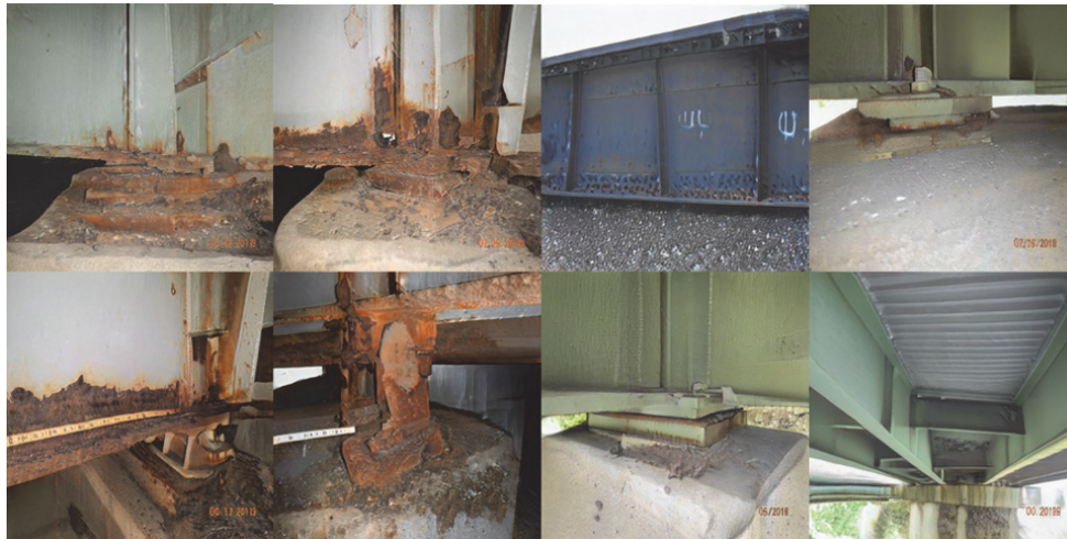
Figure 5. Examples of corrosion and non-corrosion images used for training a latent semantic boundary
