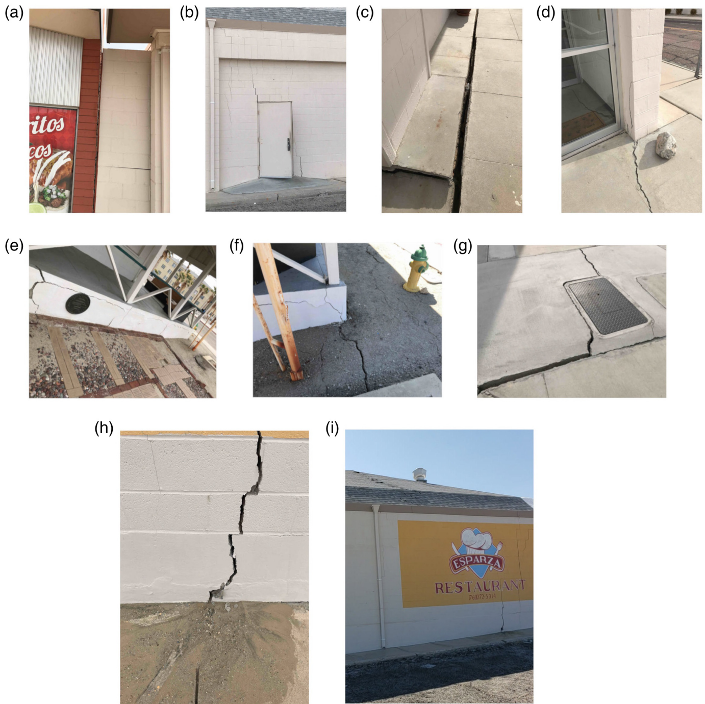
Figure 9. Ground failure effects on buildings in Trona. (a) Crack at screen wall between two buildings ( 35.75979^\circ , -117.376315^\circ ). (b,h,i) Wall cracks at the eastern side of the Esparza Restaurant with associated sand ejecta and roof damage ( 35.75957^\circ , -117.37611^\circ ). (c,d,g) Sidewalk pavement crack and offset likely from lateral spreading and ground oscillation ( 35.75982^\circ , -117.37637^\circ ; 35.75978^\circ , -117.37658^\circ ; 35.75980^\circ , -117.37606^\circ ). (e,f) Cracks in floor slab from lateral spreading and ground oscillation ( 35.759802^\circ , -117.376808^\circ ). The color version of this figure is available only in the electronic edition.
