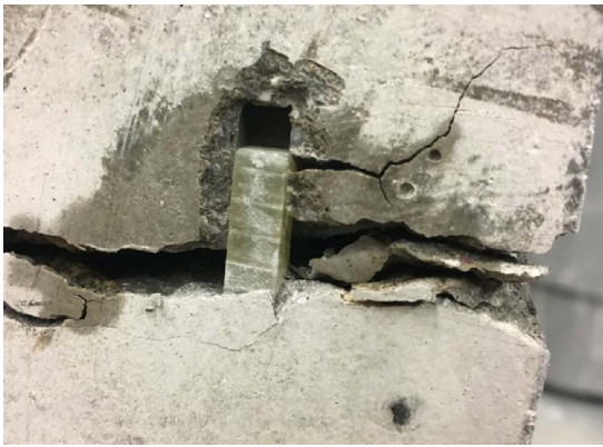
Fig. 16. A Needle in a PLN-5 beam specimen bridging a crack that has grown in width. The concrete surrounding the Needle has crumbled and spalled.
