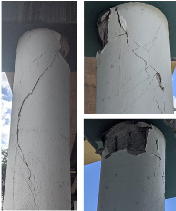
Fig. 4 Earthquake Damages to Viaduct Bridge Column in Mayagüez, Puerto Rico (source: Vidot, A. & Montejo, L.)
