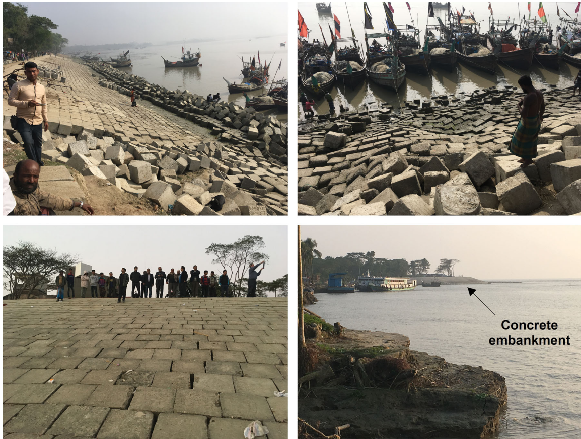
Figure 10. New embankment in Ramgati Upazila; construction started 1 February 2015 and was completed 31 January 2017.
