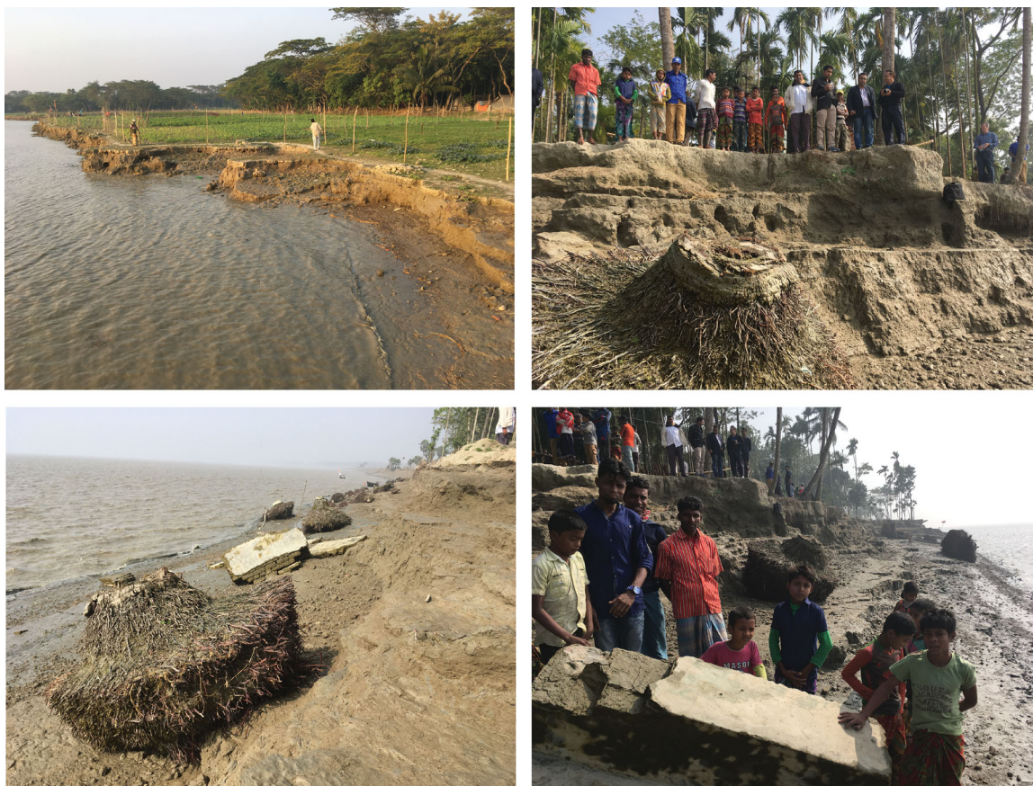
Figure 3. Shoreline change due to riverbank erosion, Ramgati Upazila, Bangladesh, January 2018.
