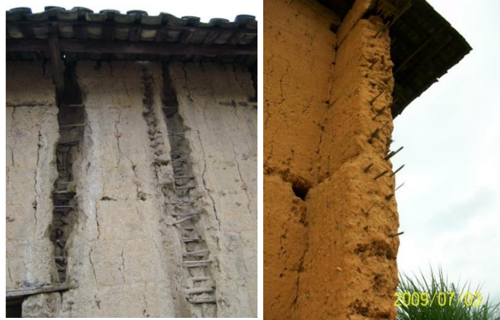
Fig. 10. Eroded earth wall exposing wooden sticks (left) and a wall section exposing bamboo strips as reinforcements (right)
