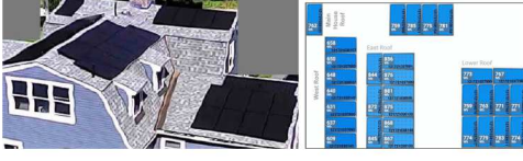
Figure 1: A residential solar array (left) with 31 panels deployed on four roof planes, and per-panel power data (right).
