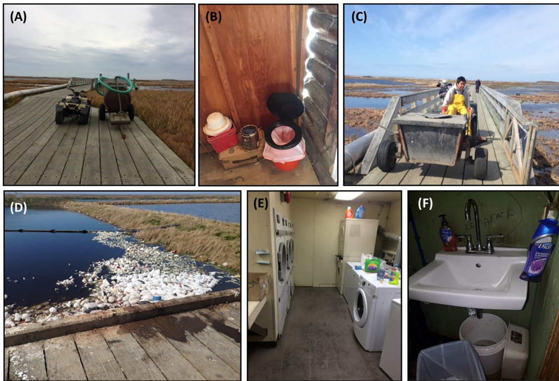
Fig. 1. Water and sanitation infrastructure in rural Alaska. (A) hauling of water using a four-wheeler, (B) honey bucket, (C) hoppers, (D) sewage lagoons, (E) community washeteria, and (F) a slop bucket for sink drain collection. (picture credits: Aaron Dotson, Kaitlin Mattos).
