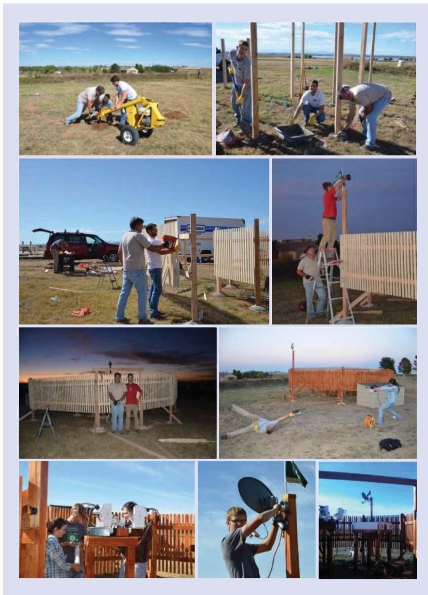
FIGURE 2. The construction of a DFIR double wind fence and the MASC and 2DVD installation at the MASCRAD Easton site (Figure 1) by members of the Electromagnetics Lab at CSU (October 2014). This kind of field construction and instrument installation project, while not entirely sounding like graduate research, and not commonly undertaken directly by university research labs, is an excellent opportunity for students to gain an appreciation of the complexity of real-world research projects as well as some broader engineering skills, advance their rapport among the group and with their graduate advisor, and strengthen the morale of the group and the project team in tackling more conventional, and presumably more difficult, research tasks. Not less importantly, as can be observed from the photos, we had a lot of fun during these sunny October Colorado days and beautiful evenings.
