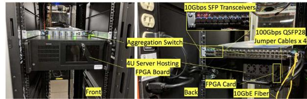
Fig. 5. Fiber Hub: aggregation switch and hosting server of FPGA pre-processor mounted on the rack shelf of networking room at WSEC.
