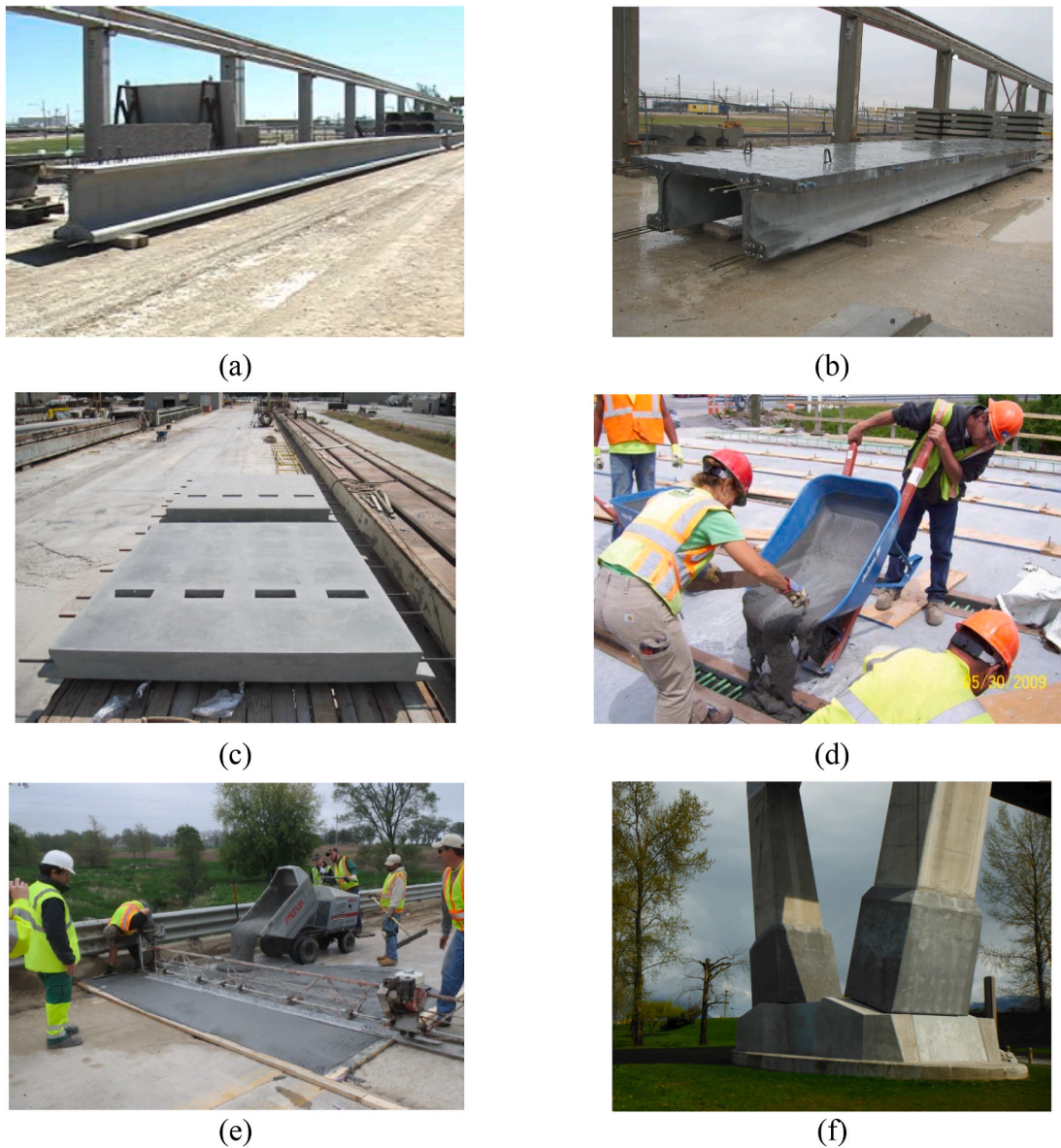
Fig. 47. Representative applications of UHPC in bridges: (a) I-shaped girder [286]; (b) Pi-shaped girder [287]; (c) precast waffle bridge deck panels [288]; (d) joint connection [289]; (e) bridge deck overlay [291]; and (f) pier jacket [293].
