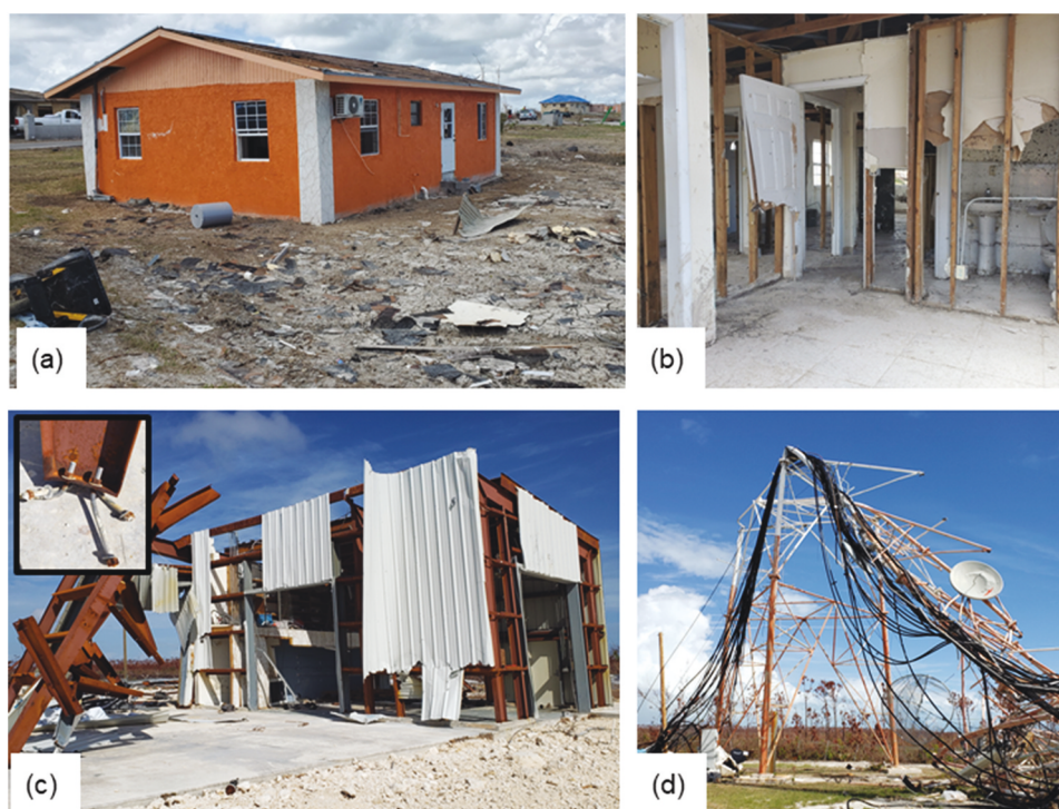
Figure 1. (a) Example of Class 1 home in Sweeting's Cay employing a mixture of lightly framed construction with a variety of sheathing materials and an annex of unreinforced masonry; (b) Example of Class 2 home near the West End; (c-d) Examples of Class 3 homes in Marsh Harbour with progressively higher levels of elevation of the primary living space.
