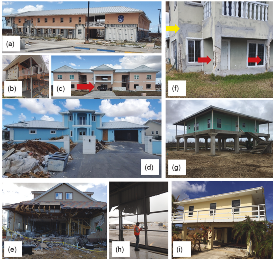
Figure 17. Freeport Metro Area (Grand Bahama Island) overview: Storm surge damage at University of the Bahamas-North campus to (a) stacked shipping container building at (26.583368, -78.570521) including (b) damage to container walls; (c) a more conventional concrete and masonry structure also sustained flood damage to its ground floor with arrow indicating spalling of concrete cover under storm surge; (d) Class 3 home with minor exterior damage but extensive interior water damage at (26.578872, -78.573360); (e) complete destruction of Class 3 home at (26.573176, -78.606356); (f) surge-induced spalling (red arrows) to concrete columns of Class 3 residence south of GBHW at (26.577974, -78.572962), with high-water mark (yellow arrow) evidencing surge inundation levels; (g) undamaged precast elevated Class 3 home at north shore of island (26.548214, -78.700064); (h) evidence of wash through at hangar at Grand Bahama International Airport (26.600281, -78.615322); (i) elevated Class 3 home in Queen's Cove, site of eyewitness surge evolution account (26.541744, -78.744403).
