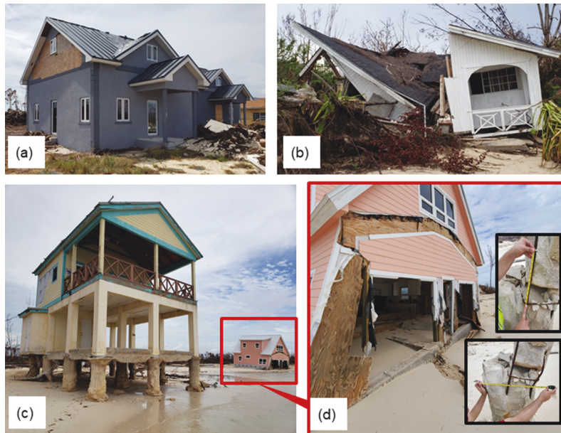
Figure 16. Varying performance levels in East Grand Bahama (Grand Bahama Island), including (a) brand new Class 2 masonry home at (26.611846, -78.354843) with minor cladding damage; (b) complete destruction of a beachfront Class 3 home in Golden Grove at (26.606874, -78.361771); Additional examples of (c) scour and (d) resulting foundation failure of beachfront Class 3 homes at (26.606950, -78.360959) and (26.614456, -78.346353), respectively.
