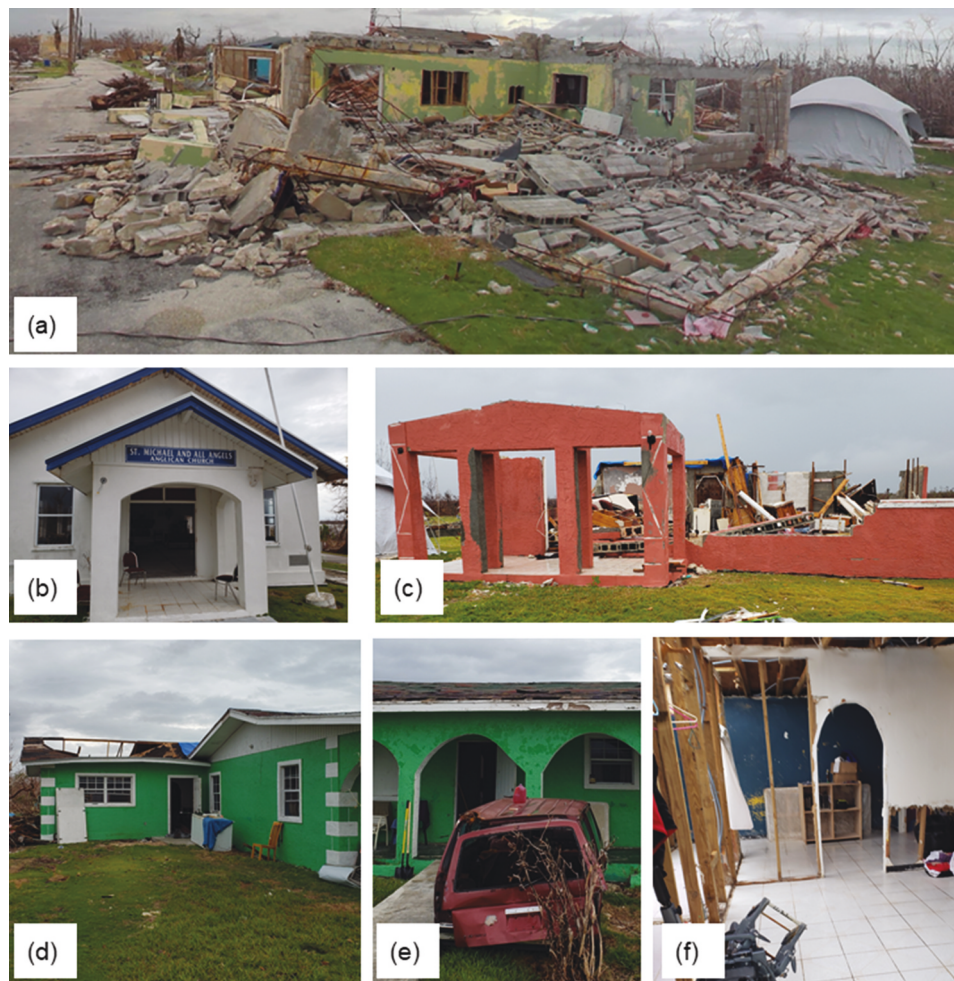
Figure 13. Sweetings Cay (Grand Bahama Island) overview: (a) panoramic image of collapsed Class 2 building; (b) St. Michael's Church at (26.609564, -77.878146); (c) complete destruction of Class 2 home at (26.609161, -77.891425); (d) well-confined Class 2 home at (26.609926, -77.877274) with (e) displaced vehicle impacting front porch column indicative of storm surge on site resulting in (f) significant interior flood losses.
