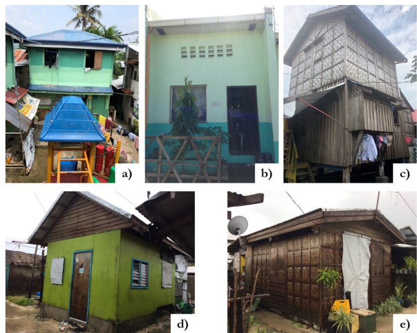
Figure 1. Photos of the studied houses, illustrating the variety of materials, shapes, and heights used: a) two-story wood house with hip roof, b) loftable masonry house, c) two-story wood house with a gable roof, d) one-story wood house with plywood walls, and e) one-story wood house with amakan walls
