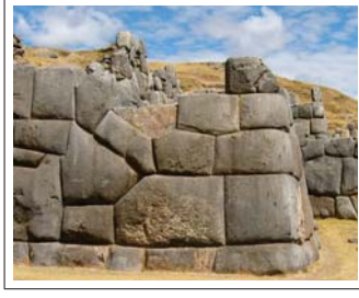
(b) Mortarless construction of an Incan wall (Bcasterline; Wikimedia).
