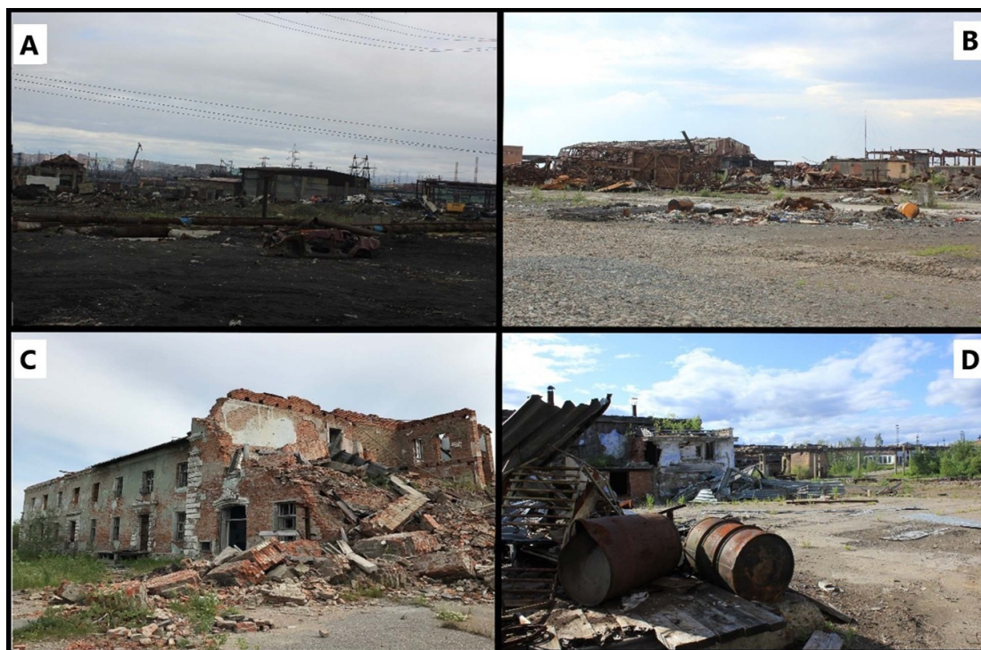
Figure 4. Examples of littered territories with abandoned and crumbling buildings: (A) and (B)—Norilsk. Photograph by A N Topoleva. Reproduced with permission. (C)—Vorkuta. Photograph by E I Bashkova. Reproduced with permission. (D)—Igarka. Photograph by A N Topoleva. Reproduced with permission.
