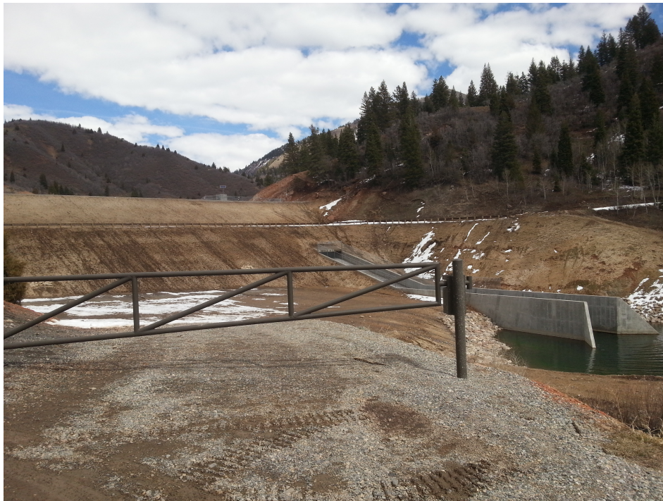
Figure 4. Tibble Fork Dam looking upstream.
