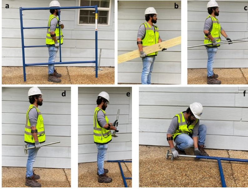
Figure 3. Shows few scaffold builder activities performed in outdoor environment (a) scaffold carrying, (b) plank carrying, (c) crossbars carrying, (d) leveling jacks carrying, (e) adjusting leveling jacks, and (f) insert leveling jacks into the scaffold
