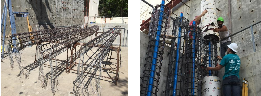
Figure 4. Rebar Cages for the three Specimen (left), Installation of Sonotube Formwork around rebar cages (right).
