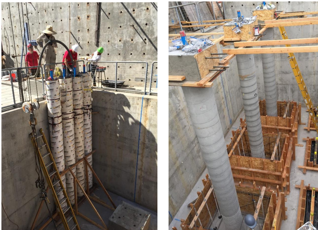
Figure 5. Concrete pour for all three rock-socketed specimens, plus one extra pile (not described in this paper), Pile placement in rock-socket formwork right before concrete placement (right)
