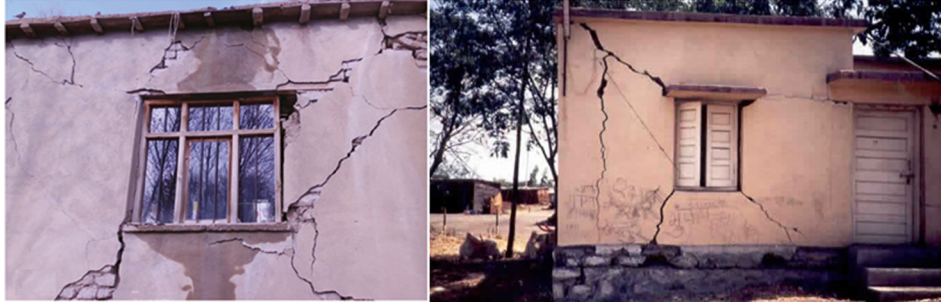
Fig. 1. Damages, in form of cracks, observed in earthen buildings due to hazard-related lateral loading.
