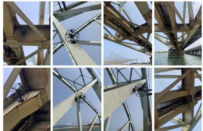
Fig. 14: Robot test on the Nam-O bridge.
