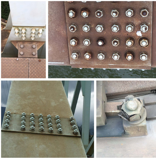
Fig. 15: Some pictures on the Nam-O bridge.
