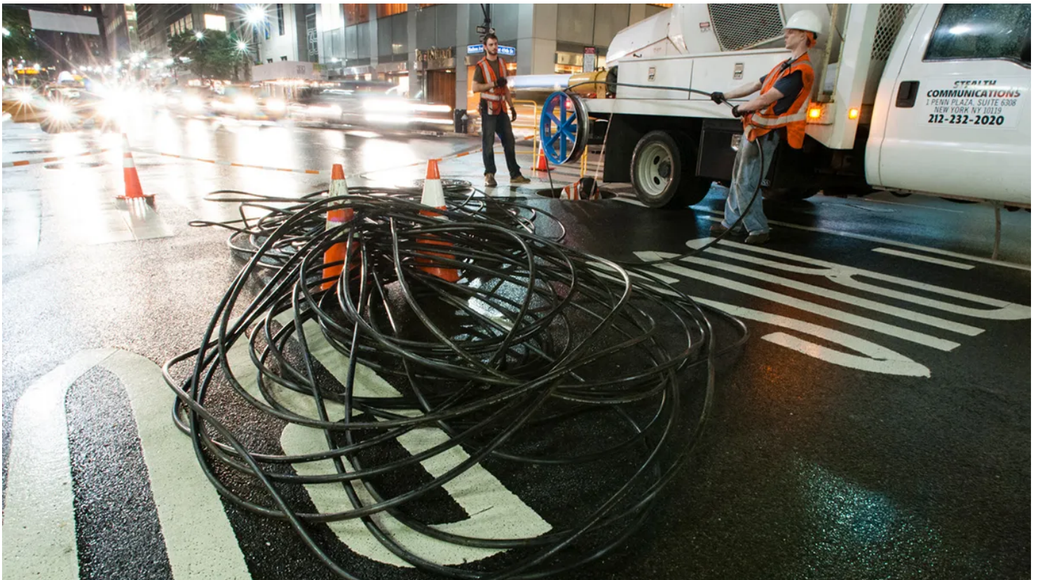
A work crew installs fiber-optic telecommunications cable under a street in midtown Manhattan in New York City. This type of cable can function as sensitive seismic strain sensors, providing Earth scientists with a deluge of data. Credit: Stealth Communications/Wikimedia Commons, CC BY-SA 3.0
