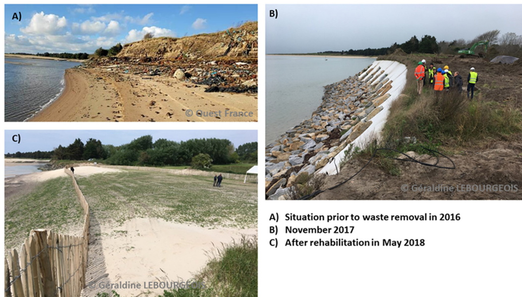
FIGURE 4 | La Samaritaine landfill (A) prior to waste removal in 2016, (B) during waste excavation (November 2017) with erosion being stopped by riprap and a geotextile, (C) the restored site (May 2018). Photography (A) courtesy of Ouest-France archives, (B,C) courtesy of Geraldine Lebourgeois/La Presse de la Manche.
