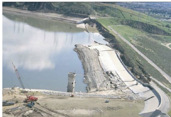
Figure 2. Lower San Fernando dam after the San Fernando earthquake (1971) (Courtesy of the National Information Service for Earthquake Engineering, EERC, University of California, Berkeley)
