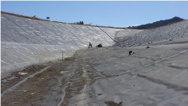
Fig. 2. Exhumed liner system.
