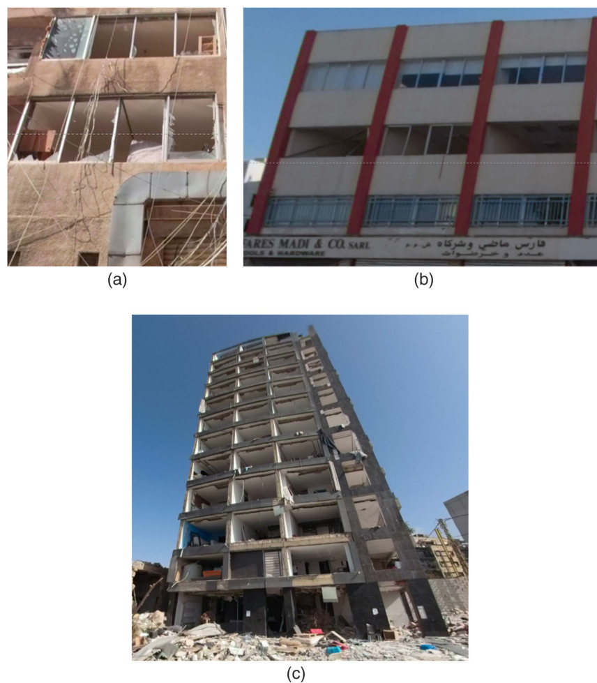
Fig. 14. Façade damage levels: (a) Wxx-1, damage to windows only; (b) Wxx-2, damage to windows and frames; and (c) Wxx-3, complete blow-out of panels within building frames.
