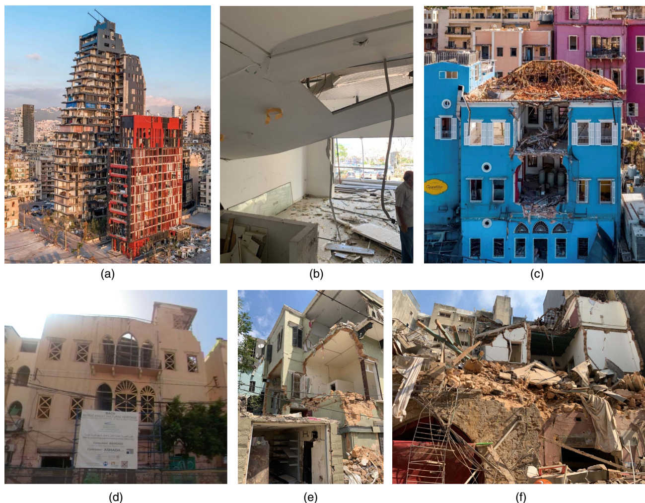
Fig. 13. Buildings with variable levels of blast damage: (a and b) RC structures with moderate nonstructural damage (e.g., cladding, false ceilings) but no apparent structural damage (D2); (c) stone masonry building with heavy damage (D3) including significant cracking of exterior bearing walls, failure of façade arches and balconies, and partial roof collapse; (d and e) partially collapsed stone masonry buildings (D4) (image reprinted from Sadek et al. 2021a); and (f) totally collapsed stone masonry building (D5). [Images (a and c) by Rami Rizk; images (b, e, and f) by Mayssa Dabaghi.]
