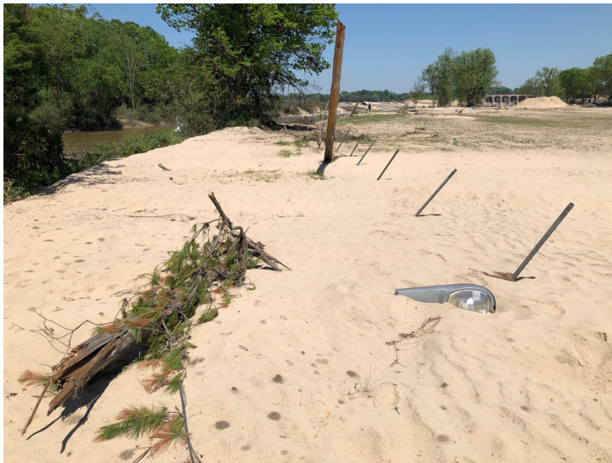
Figure 7: Burial of light post beneath sand deposits from flood water
