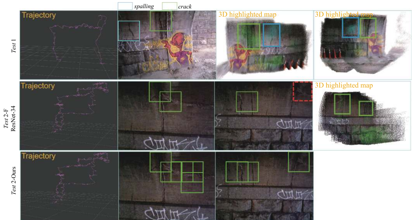
Fig. 10. Two automotive field tests, Test 1 and Test 2 , are carried out using CityFlyer. In both tests, we illustrate the drone's trajectory, region detection results, and the 3D reconstructed mapping with defect highlighting.
