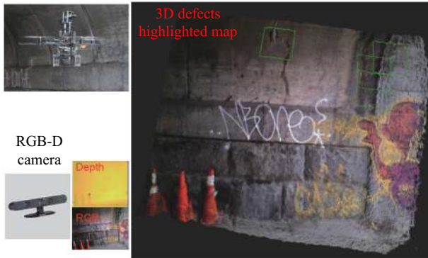
Fig. 1. Illustration of our robotic inspection system, it is developed based on the CityFlyer quadrotor robot aiming to perform the concrete structure inspection. The right side image shows the inspection result that we got under a bridge located at Riverside Drive & West 155th Street, New York. The robot is equipped with an RGB-D camera which is used for localization and 3D mapping with defect visualization.
