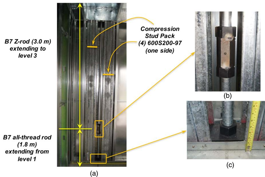
**Fig. 3.** Tie-down assembly details of the Level 2 corridor shear wall: (a) overall view; (b) coupler and double-nut connection; and (c) bearing plate and washer connection (embedded into the bottom track). (Images by Xiang Wang.)
