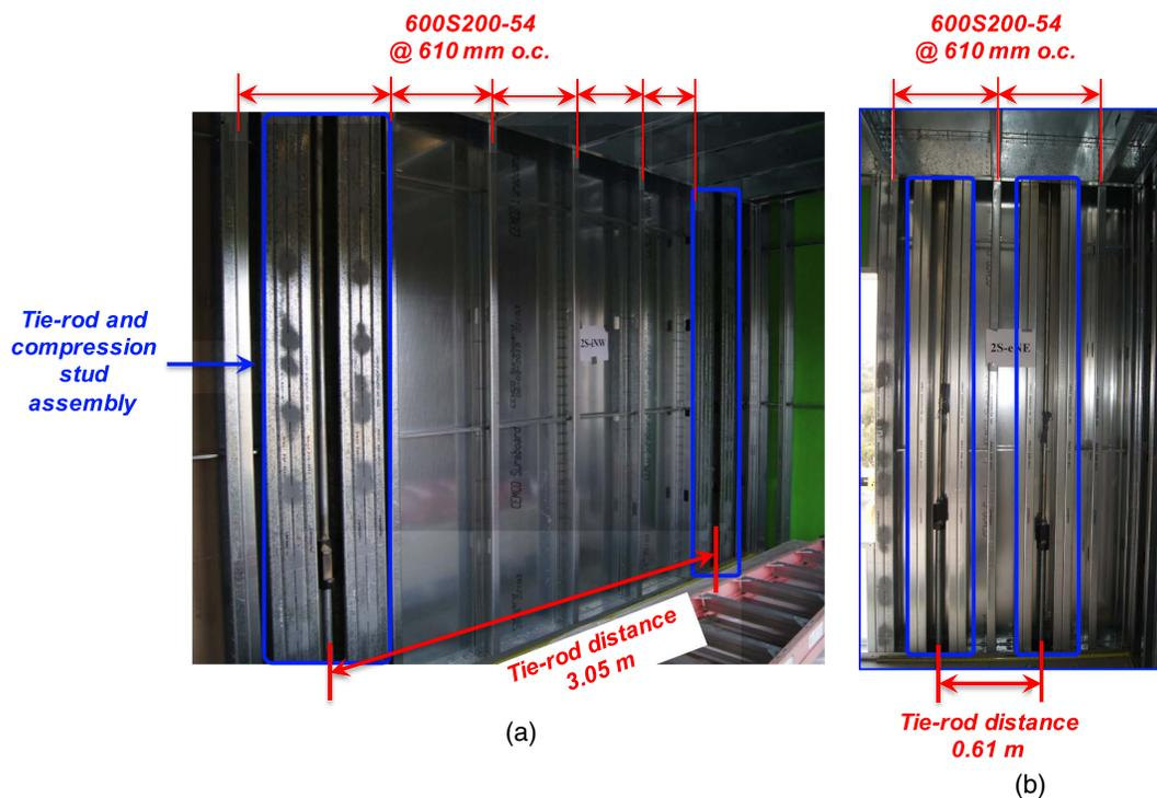
**Fig. 2.** Shear wall framing at Level 2: (a) corridor shear wall (west segment) (adapted from Hutchinson et al. 2021, © ASCE); and (b) longitudinal corner shear wall (northeast segment) (image by Xiang Wang).
