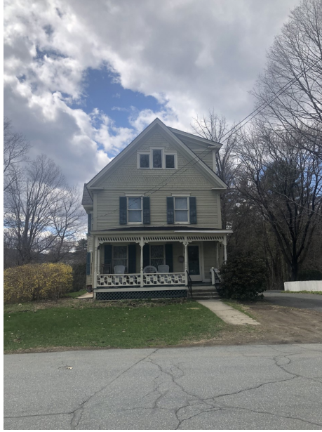
Figure 6.1: Experiment 1 Testing Site. A residential house was used as a smart home environment.
