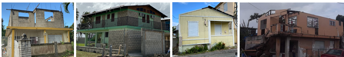
Figure 2. Photos of Puerto Rican informally-constructed houses [Photos: Polly B. Murray and the authors]
