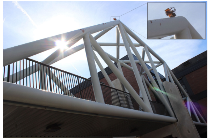
Fig. 19. The robot operates on a cylindrical steel bridge to perform thickness measurements and checking for corrosion.
