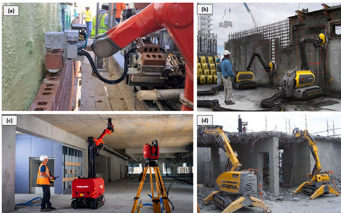
Fig. 8. Examples of application of robotics in building construction: (a) Architecture-related, façade installation [120]; (b) Structure-related, shotcrete for shear walls [121]; (c) Interior layout-related, BIM-enabled mobile ceiling-drilling robot [122]; (d) Demolition of buildings and existing structures [123]
