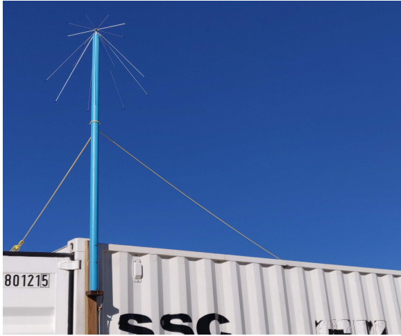
Fig. 4. A photo of the SPUTNIK discone and electromagnetically compliant (EMC), shielded structure in the Karoo. The discone is mounted atop, but electrically-insulated from, the structure.
