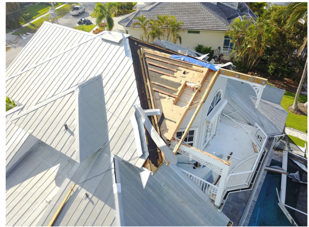
FIGURE 7 | UAVs with high-resolution cameras are well-suited capture perishable data (e.g., roof cover damage, debris field), and provide complementary datasets for ground-based damage surveys. The areal perspective of UAVs reveals structural damage that is hidden from the view of ground-based damage surveyors. Photograph by Kwasi Oerry was acquired under sponsorship from the Florida Building Commission.
