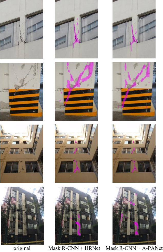
Fig. 10. Prediction of Mask R-CNN with Attention PANet and HRNet for 2017 Mexico City earthquake images [33].
