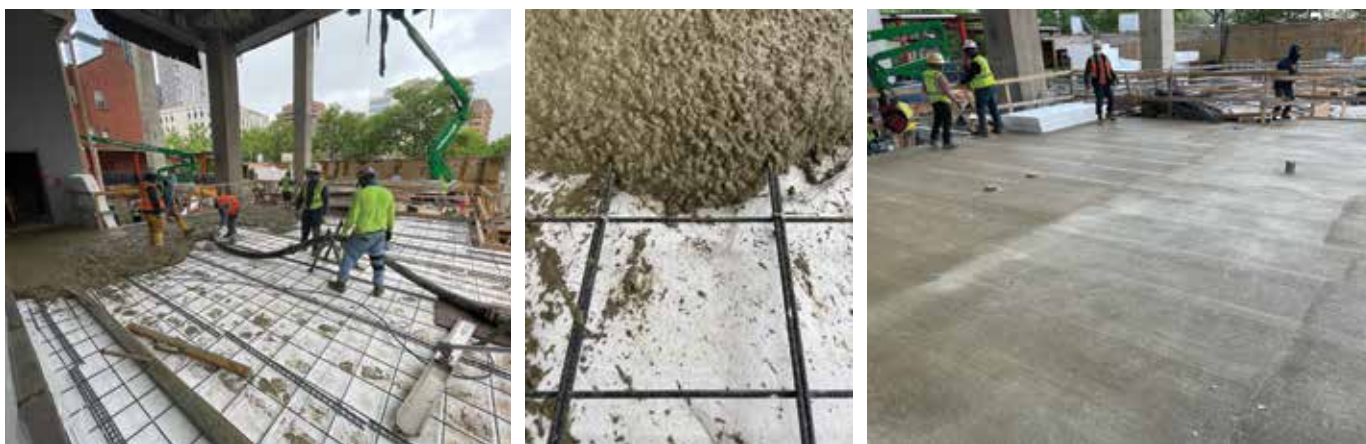
Fig. 5: Concrete placement for one of the topping slabs
