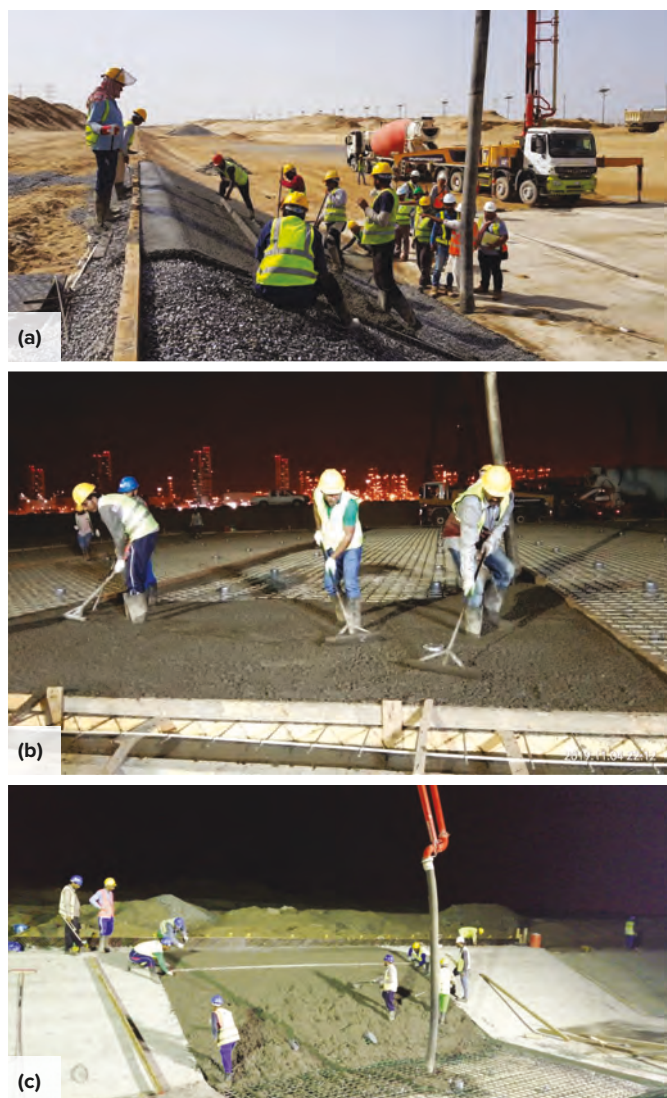
Fig. 8: Concrete placements at the JEC-FMC: (a) blinding layer in the sloped side; (b) a panel in the base slab; and (c) a panel at a sloped side
