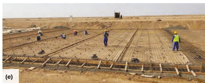
Fig. 6: The base slab was reinforced with grids of GFRP bars: (a) delivery of bars; (b) storage of bars on the blinding layer of an interior panel of the base slab (note openings in the blinding layer for later installation of weep hole pipes); (c) initial placement of bars; (d) grid assembly; and (e) final preparation of bar grid and longitudinal joint formwork
