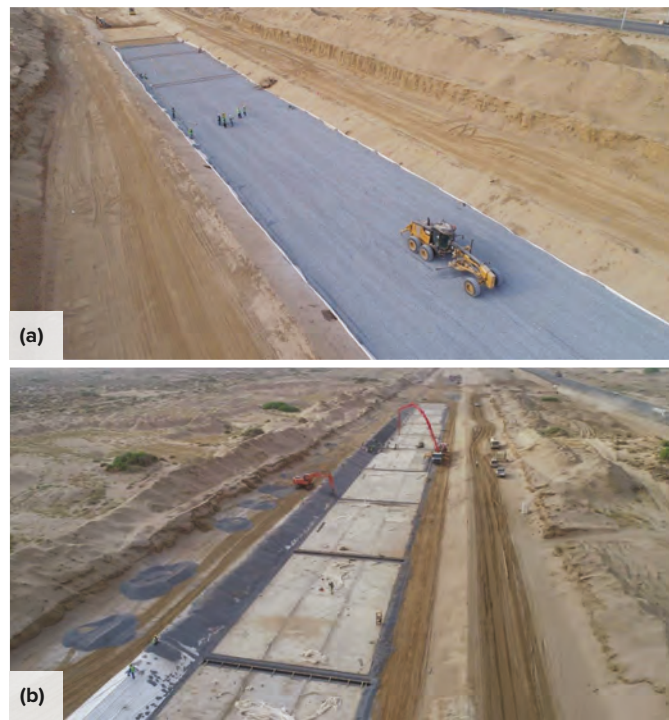
Fig. 5: Placement of the drainage layer: (a) for the base slab; and (b) for the sloped sides. The drainage layer for each of the sloped sides of the channel was placed after completion of the blinding layer for the base
