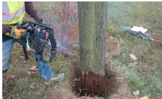
Figure 2. Conventional wooden utility pole inspection method.
