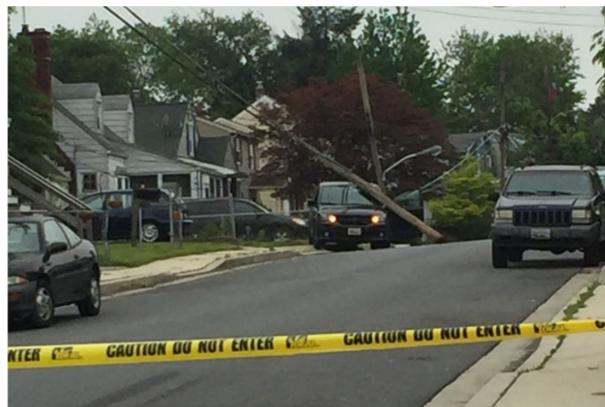
Figure 1. Accident of a wooden utility pole failure in Baltimore in 2019.
