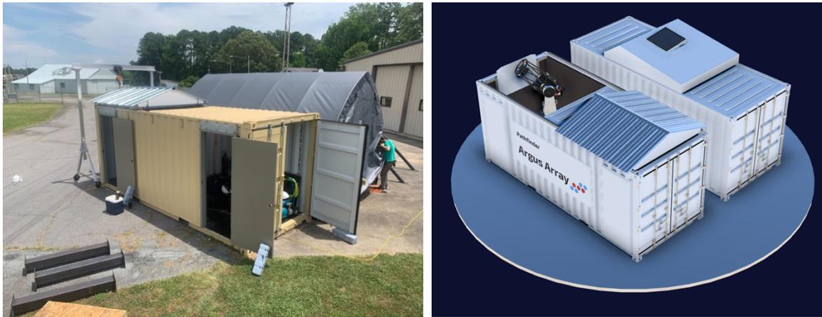
Figure 6: *Left:* The Pathfinder enclosure under construction in Chapel Hill, NC as of June 2022. The Service Module is in the foreground and the ArgusSpec Module sports a retractable roof. The Optics Module is beneath the tent. *Right:* Exterior view of the completed Pathfinder enclosure in similar perspective as the left image. ArgusSpec is visible with roof retracted. The Optics Module is in the background showing the window cupola. Sunshield not shown.
