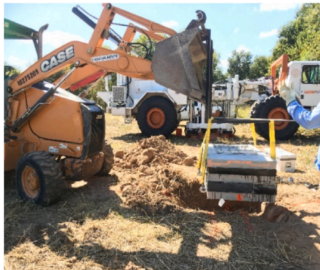
Fig. 3. Installation of periodic foundation.
