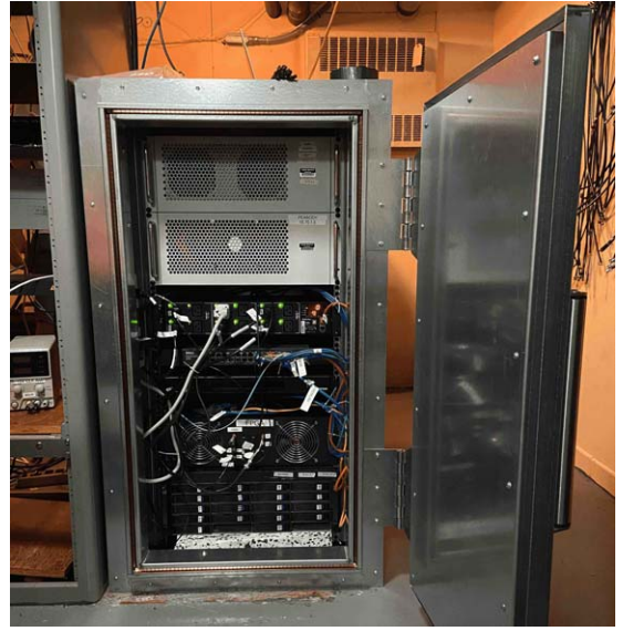
Figure 5. RF-shielded rack located in the main control room at ARO. The rack includes (from top to bottom): controller node, analysis node, power distribution unit (PDU), main switch, GPS unit, ICE/FPGAs, and recording node.
