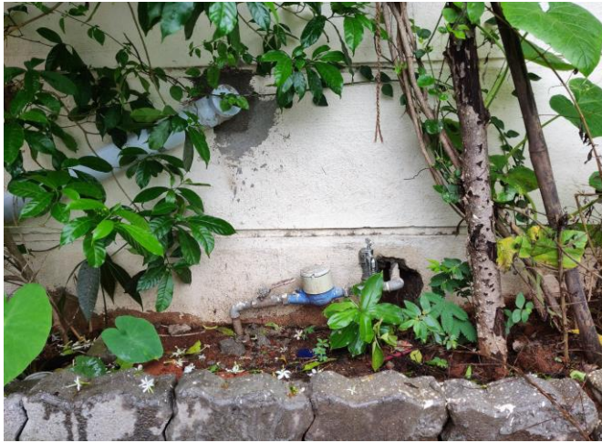
Fig. 3. Existing, older metered water connection in some areas. These meters are either dysfunctional or connected to a very limited number of households. The meters were introduced around the year 2000 but were retracted due to technical issues and were a failure (Image source: Lead author. Information Source: participant 8).
